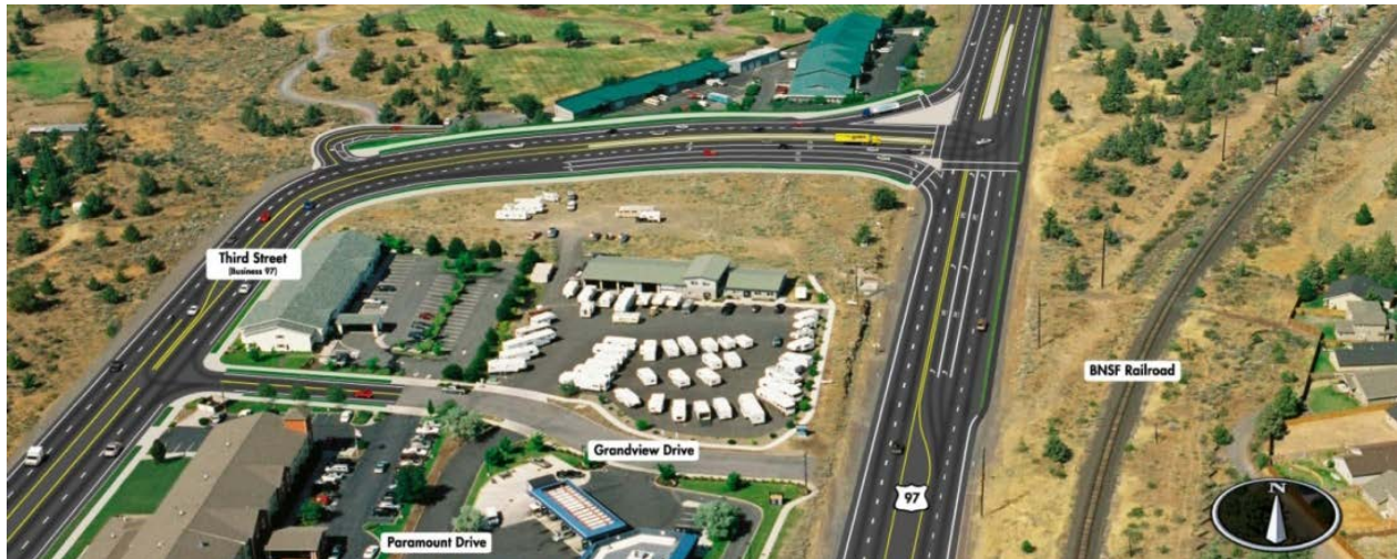
Figure 7: Existing US 97 will be converted into a business route for local traffic, connecting to the new alignment of US 97 north of Bend.
