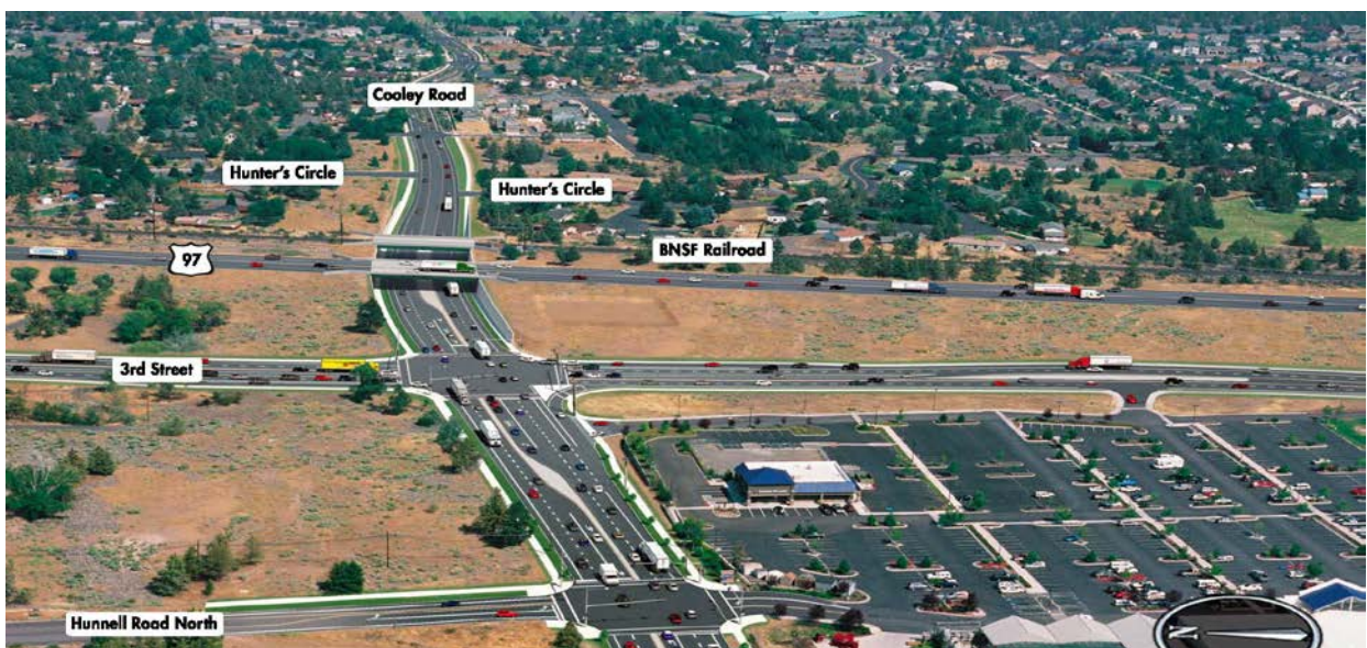
Figure 8: Cooley Road grade separated from US 97 and BNSF Railway.
